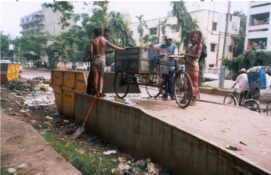
Photo 3: Ramped transfer point in Bangladesh (Jonathan Rouse)
